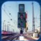
1 Trackside traffic control box Signal lights box
